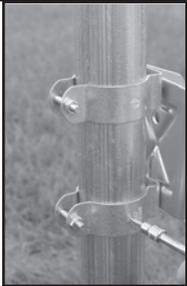
3. Now place clamps on pole and bolt onto pole. Screw the (2) self-tapping screws through the clamp and into pole on each side of the clamp (this will eliminate the twisting of the winch when in use).
