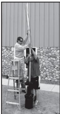
9. Using a ladder and a helper, place the remaining pole sections atop the standing sections. Be sure to allow both ends of the rope to dangle close enough to the ground that they can be reached easily.
