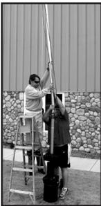
8. Using a ladder and a helper, place the two remaining pole sections atop the standing sections.
